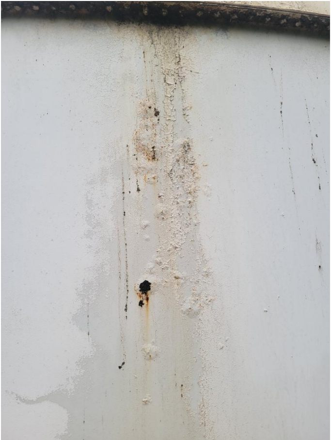
Panel Damage - Repair attempt on July 17th
