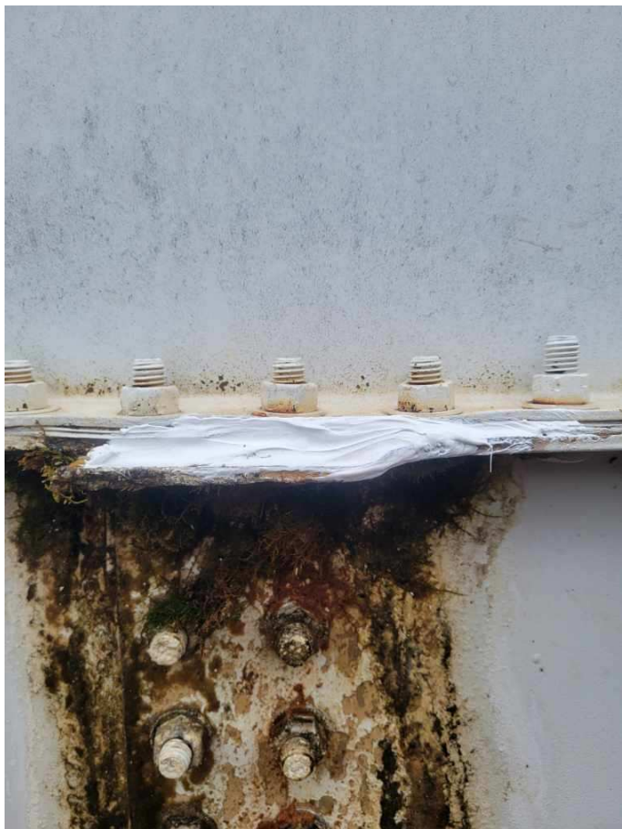
Panel Damage - Repair attempt on July 17th
